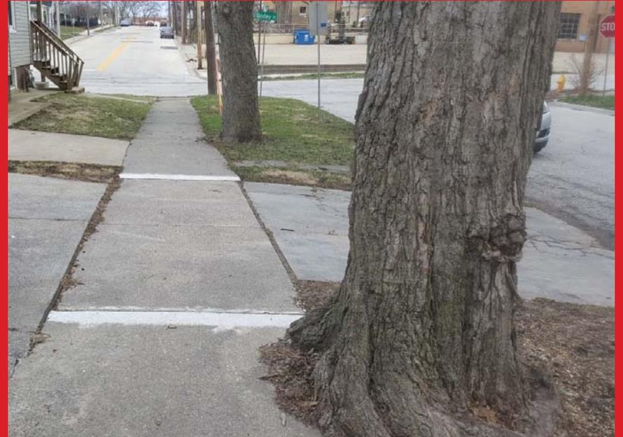
Grinding 2 panels: Each grind was 5 feet wide, 3/4 inch high = 7.5 inch-feet total. \$277.50 under proposed Grind contract. Replacement of the 2 5X5 panels (50 SF), 4" concrete = \$475 under proposed Sidewalk contract.
