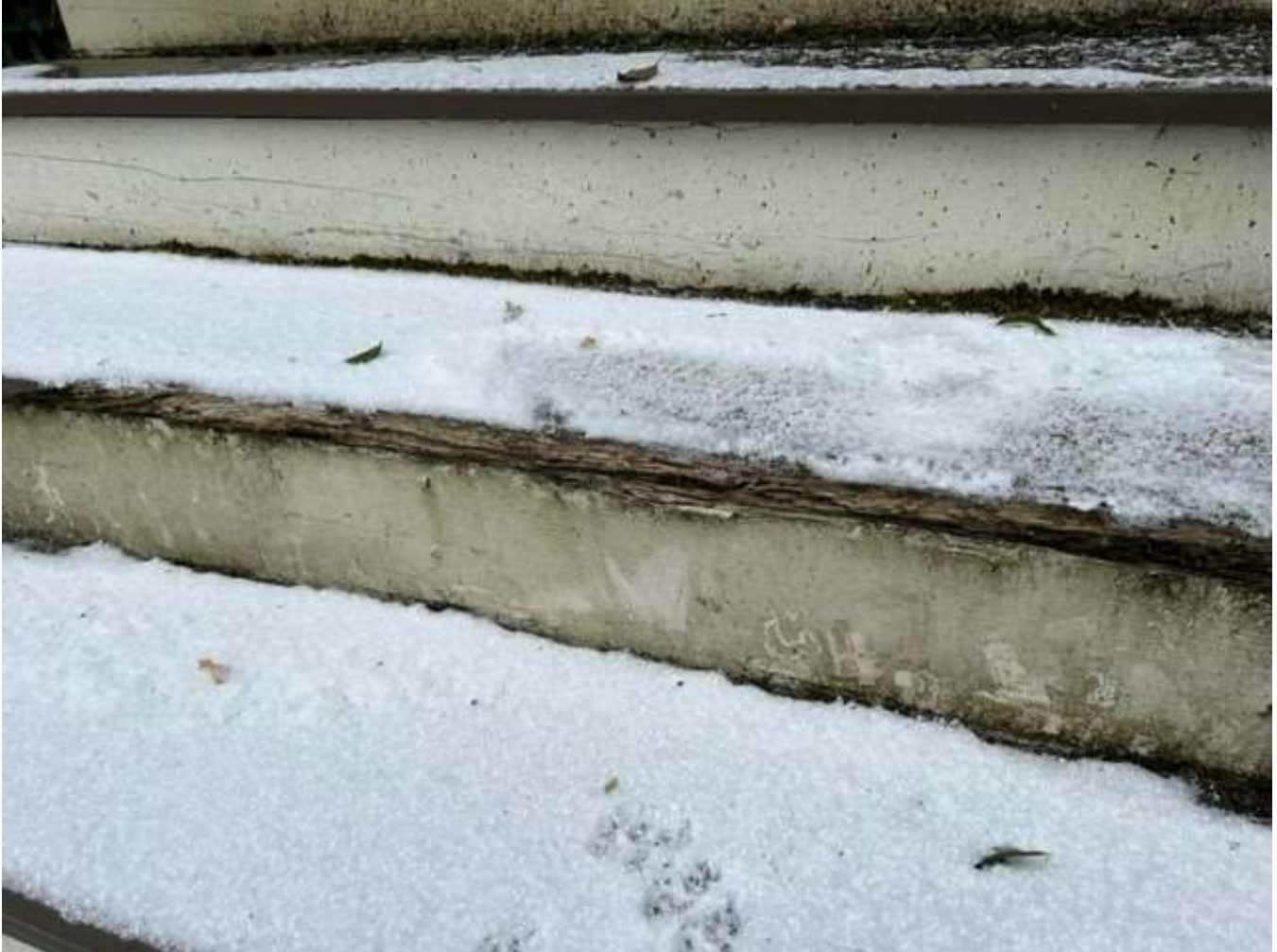
Main Porch Stairs
