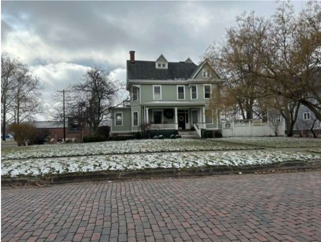
Above: The subject property at 905 E. Jefferson Street
